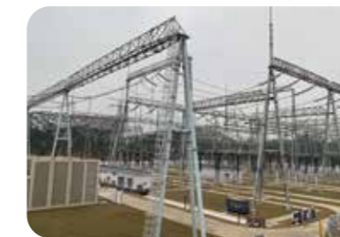
Electricity power inspection
